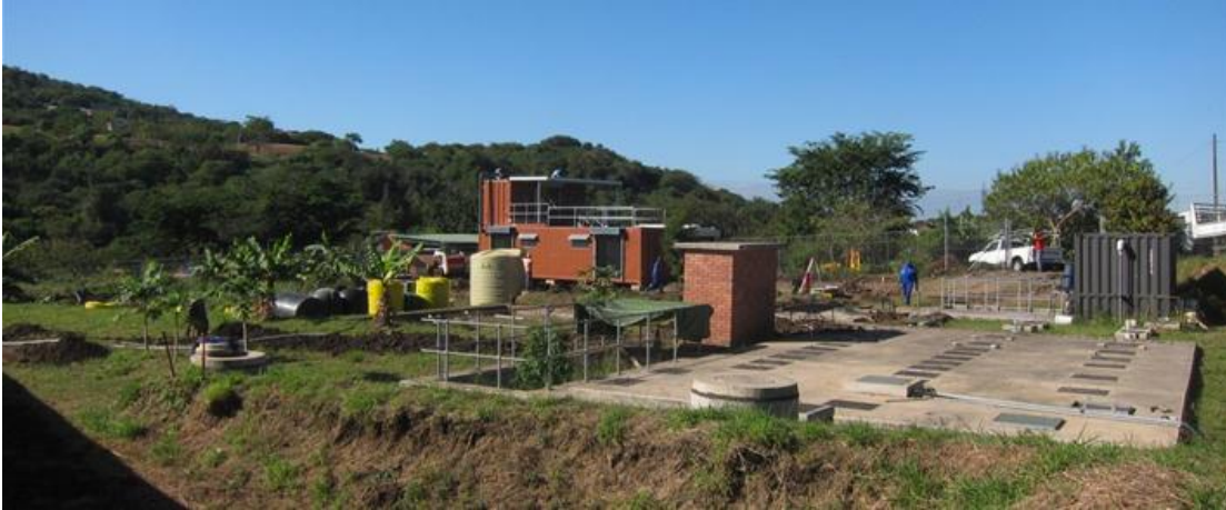
Figure 18: DEWAT trial plant
