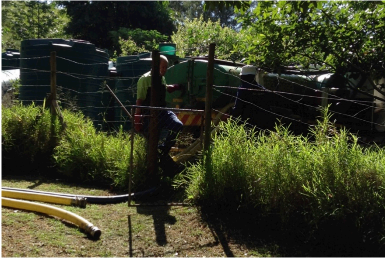
Figure 14: Vacuum tanker in place for septic tank emptying
