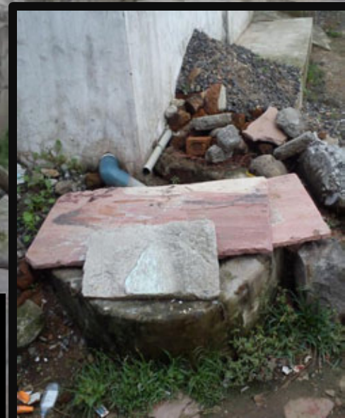
Community Septic Tank connected to households via chambers. (Dewas, M.P)
