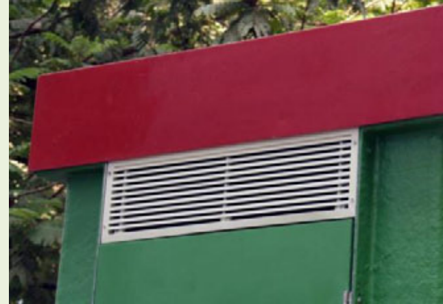
Louvers at top position of the shelter
