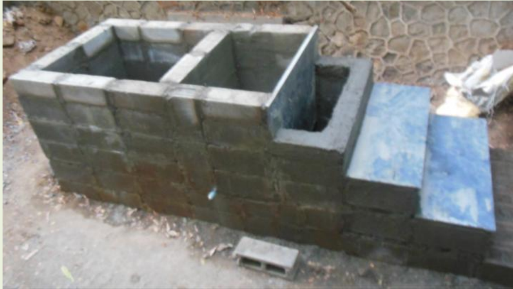
Completed pits, ready for further toilet pan assembly
