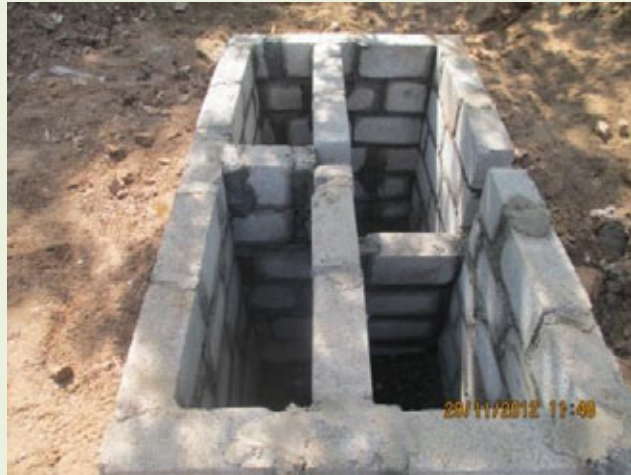
Pits under construction
