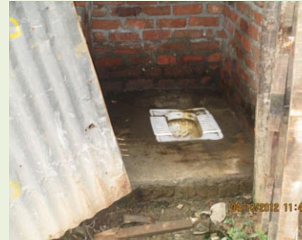
Contractor Labour colony toilet, IITB
