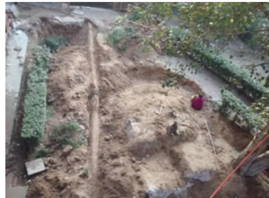
Excavation at the site
