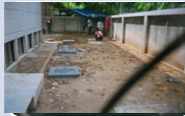
Anaerobic Baffled Reactor (Secondary Treatment)
