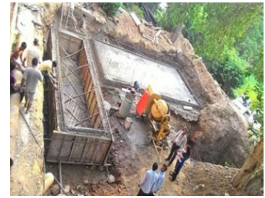
Construction at the site
