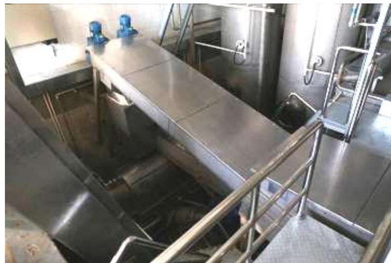
Separation, sand removal, pyrolysis device
