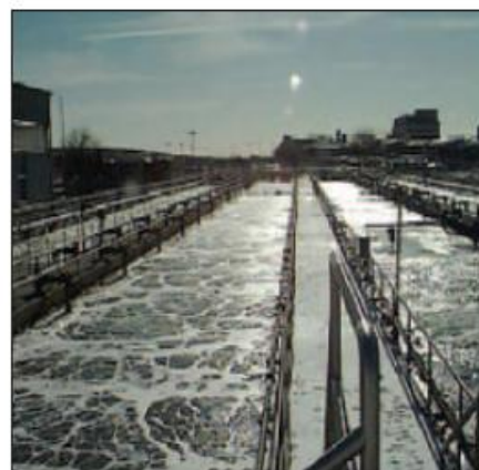
View of Centrate Tank at 26th Ward WPCP
