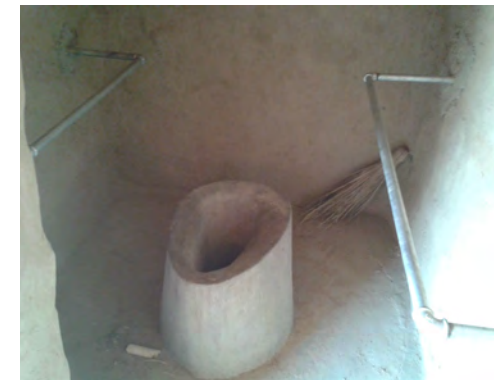
Fixed toilet seat with handrails. Rails could be made from wood to reduce cost.
