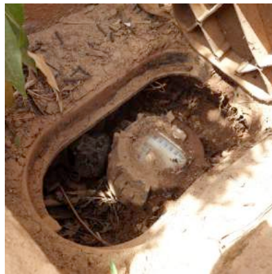
Centralised example: Connection to water-supply network
