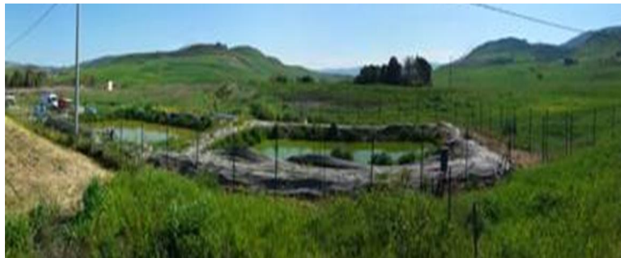
Horizontal Subsurface CW (H-SSF)+ lagooning + storage reservoir
