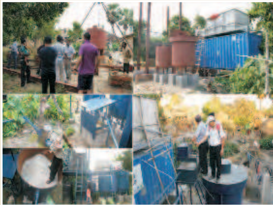
Construction of Groundwater Scheme-Eco-ndia Project
