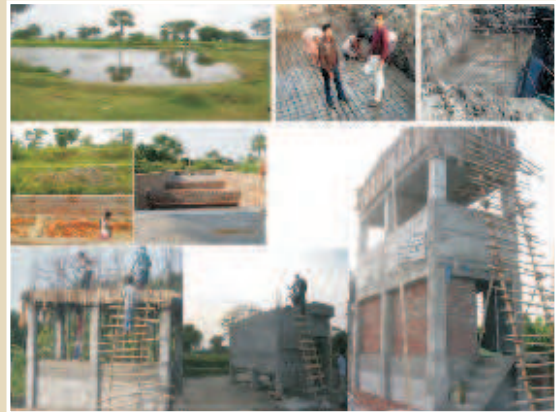
Construction of surface water scheme-Eco-India
