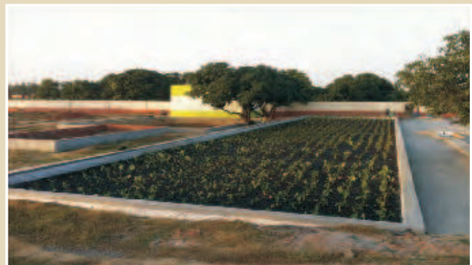
Horizontal Flow Constructed Wetlands SWINGS Project
