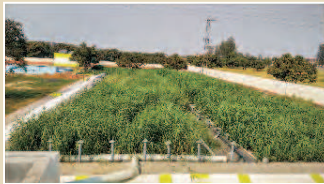
Vertical Flow Constructed Wetlands-SWINGS Project
