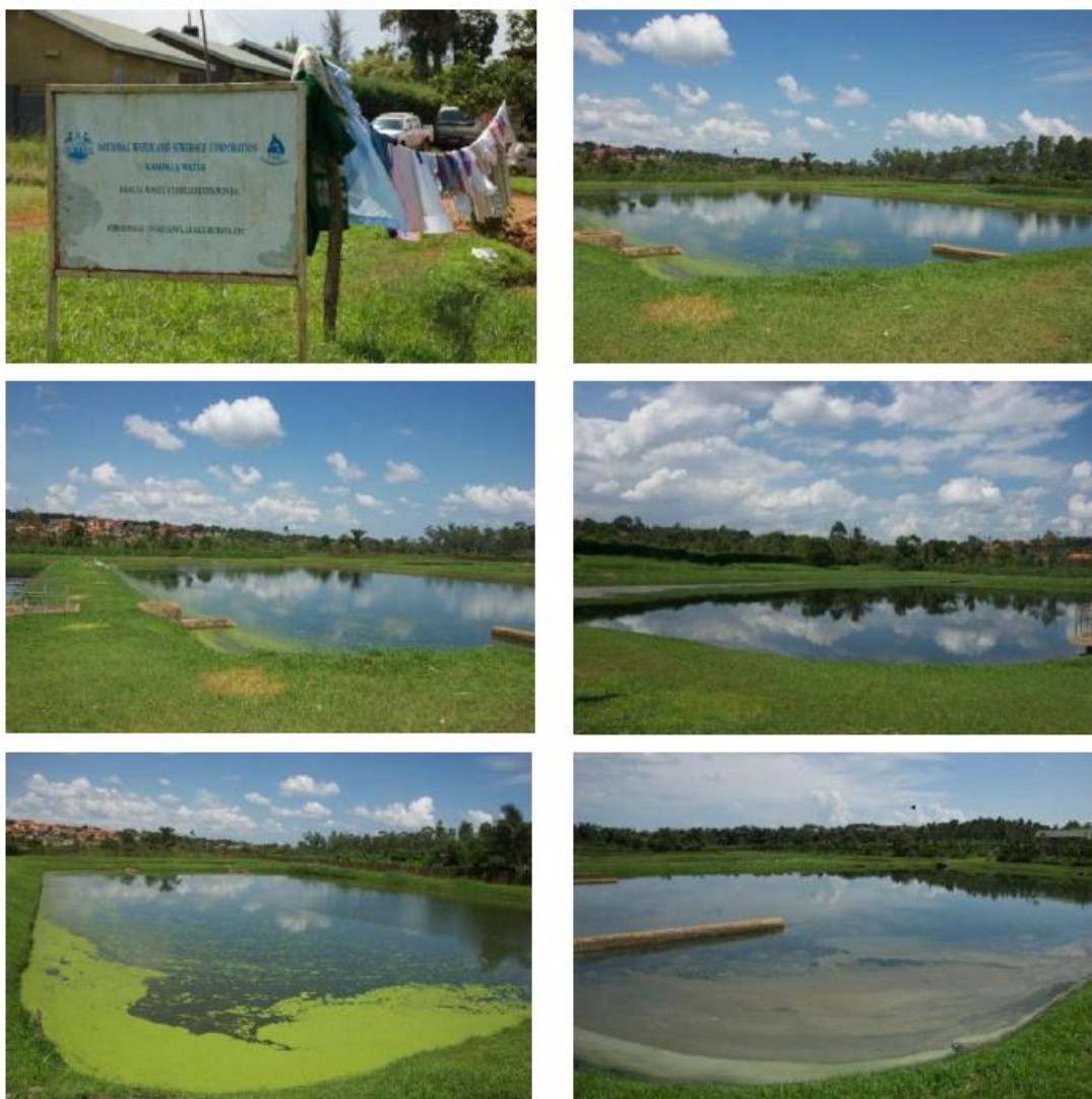
Figure 10: Waste stabilization ponds in Naalya, Kampala. Photos: Lars Schoebitz, November 2013.
