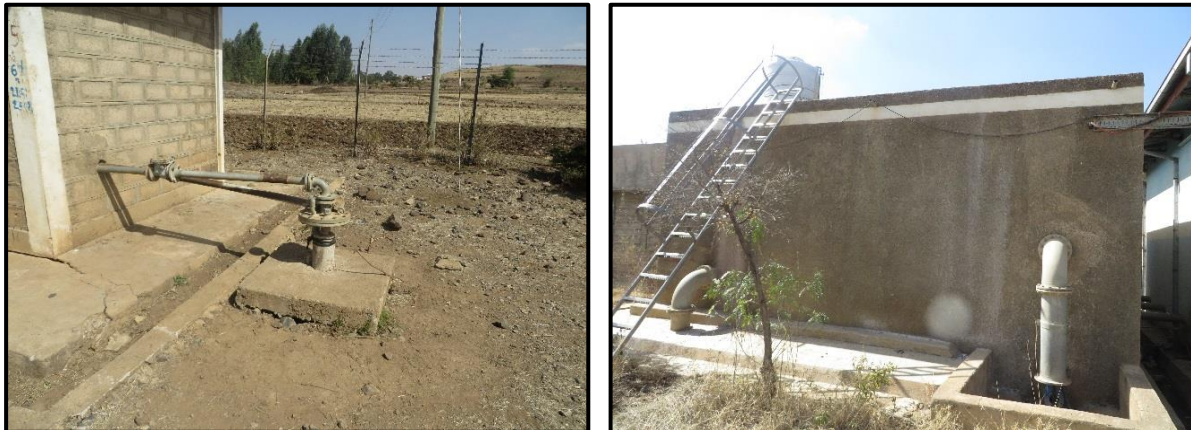
Figure 8: a) Groundwater well. b) Water reservoir provided with a chlorine dispenser (photo credit: Oscar Veses).
