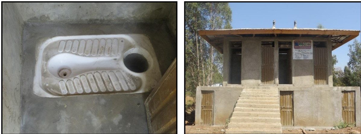
Figure 7: Inside and outside of an EcoSan in a public school (photo credit: Oscar Veses).
