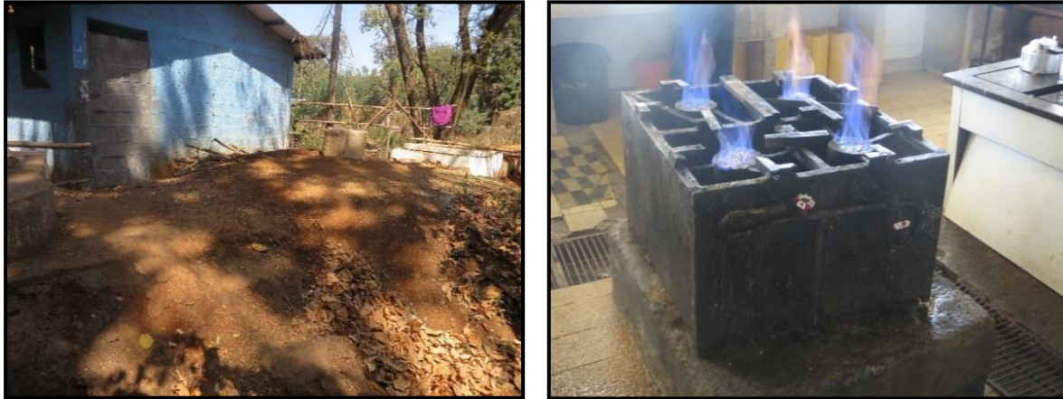
Figure 8: a) Bio-digester covered in soil. b) Biogas used for cooking purposes in the Felegehiwot referral hospital (photo credit: Oscar Veses).
