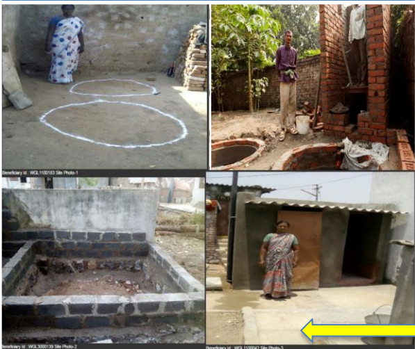
Different stages involved in construction of toilet
