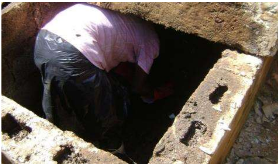
Figure 22: These workers have entered the pit without a mask or protective jacket, putting themselves at unnecessary risk of infection in order to more easily remove the sludge. When they climb out of the pit their boots will track sludge around the household environment, into the vehicle and into their home, putting others at risk of infection as well.
