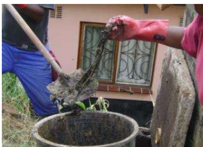
Figure 12 A worker handles trash in the sludge directly with her hands, heavily soiling her gloves.
