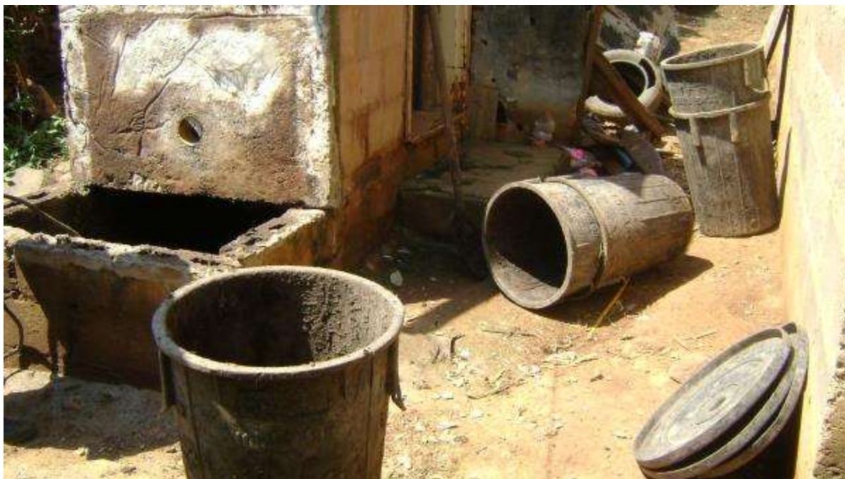
Figure 26 In the cramped conditions at many sites, the presence of numerous grossly contaminated bins represented a large potential contamination “footprint” at the site. Workers carried with them no barriers on which they could place the bins to protect the earth.
