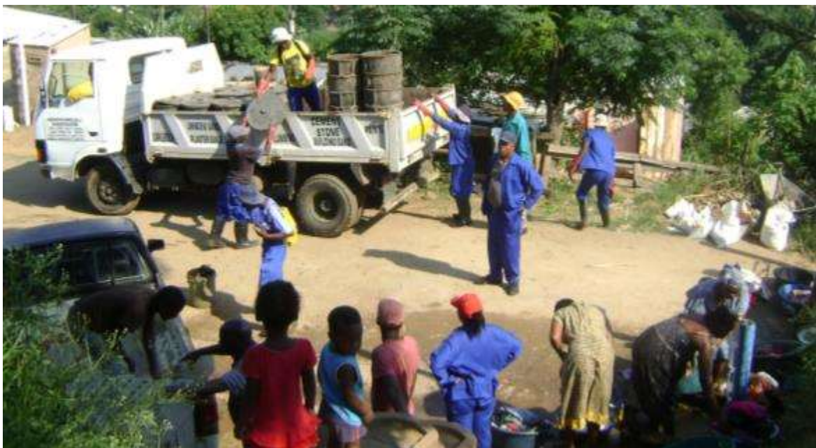
Figure 31 A vehicle from a local hardware was hired to transport the bins to the disposal site. Several people from the community passed through the area where sludge was loaded or empty bins off loaded. Potential contamination of the vehicle (as well as the environment) can be seen from workers' gloves, boots and the contaminated bins.
