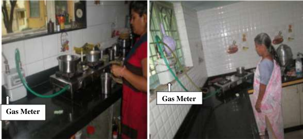
Photos 12 -13 Gas meters attached to gas burners used for cooking
