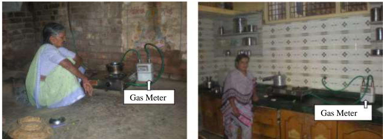
Photos 14 -15 Gas meters attached to gas burners used for cooking
