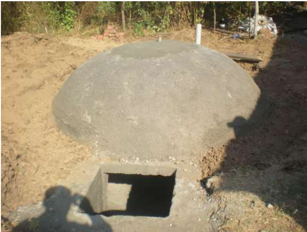
Photo 10 Complete biogas plant with Inlet tank and outlet chamber under construction
