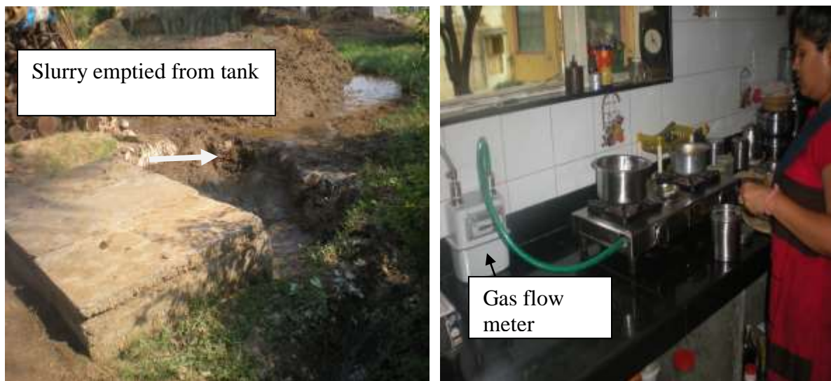
Fig 2: Slurry from a Toilet linked biogas plant Fig 3: Use of biogas for cooking
