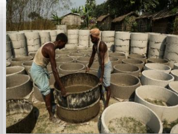
Cement ring manufacturing
