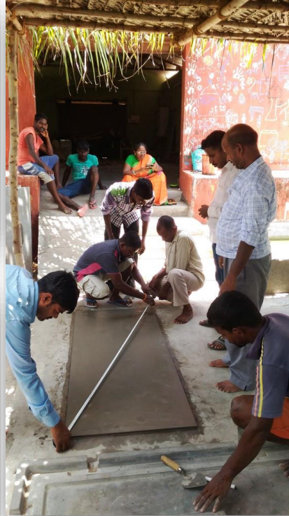
Mason training on toilet construction
