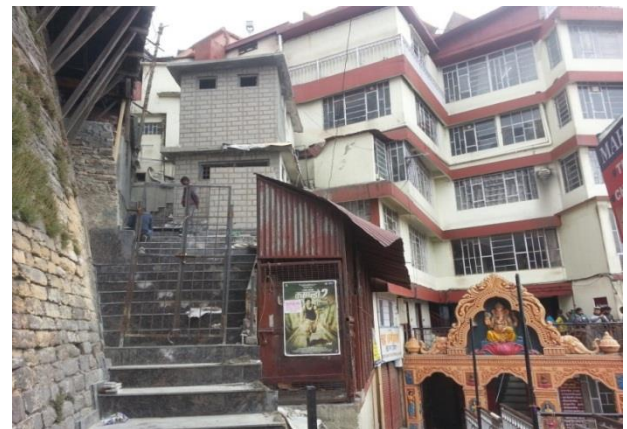
Pic: Rehabilitated Public Toilet @ Ram Mandir, Shimla
