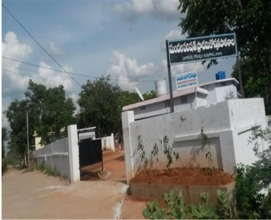
Front view of the school and premises
