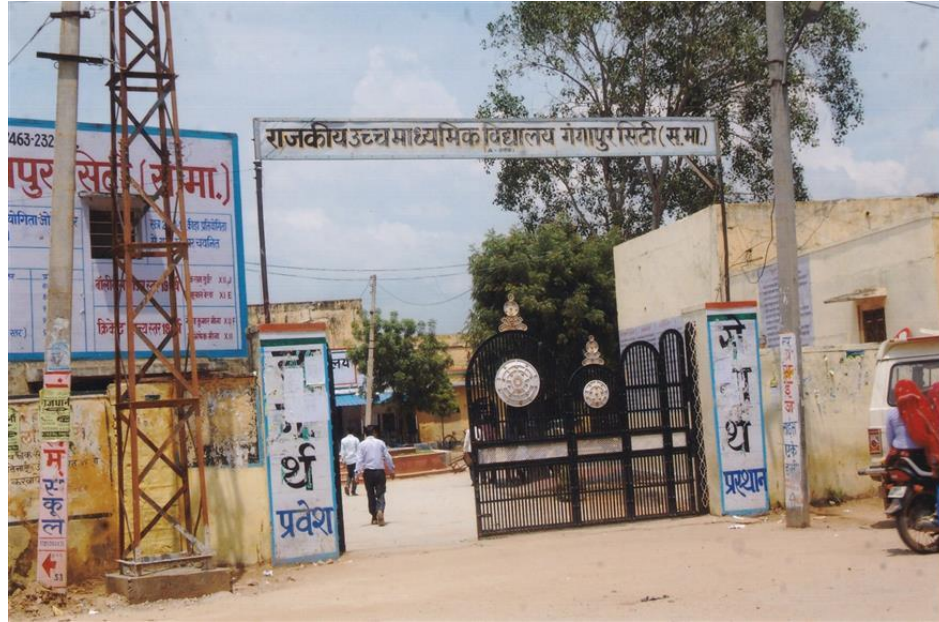
Front view of the school and premises
