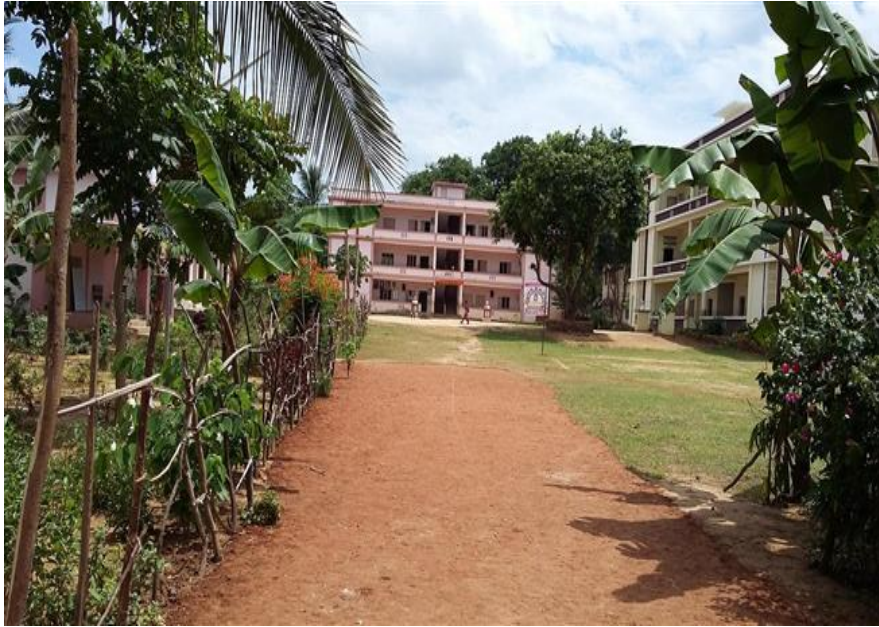
Front view of the school and premises
