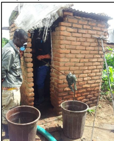
Figure 5-4 Fishing of rubbish during desludging of household latrine
