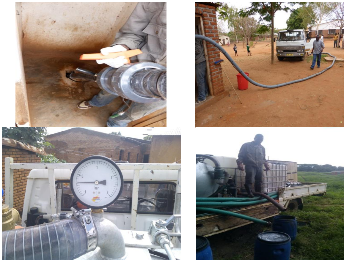
Figure 3.7 Pumping out faecal sludge and emptying in 50 L containers
