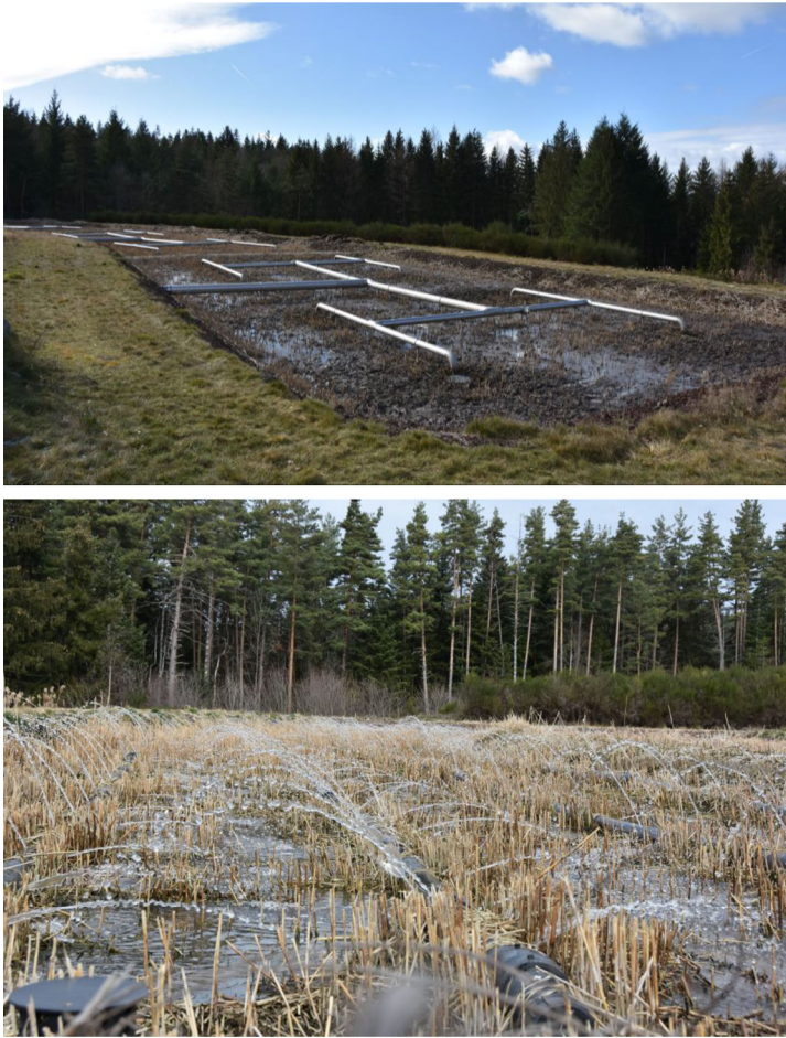
Figure 5.4 Distribution of wastewater French VF wetland; top: first stage; bottom: second stage. Photos courtesy of Pascal Molle.
