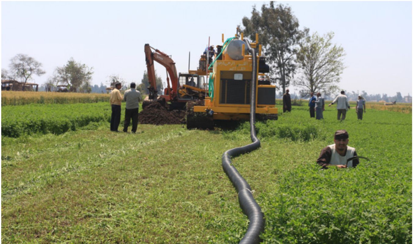
Subsurface drainage network used to control the groundwater level and soil salinity
