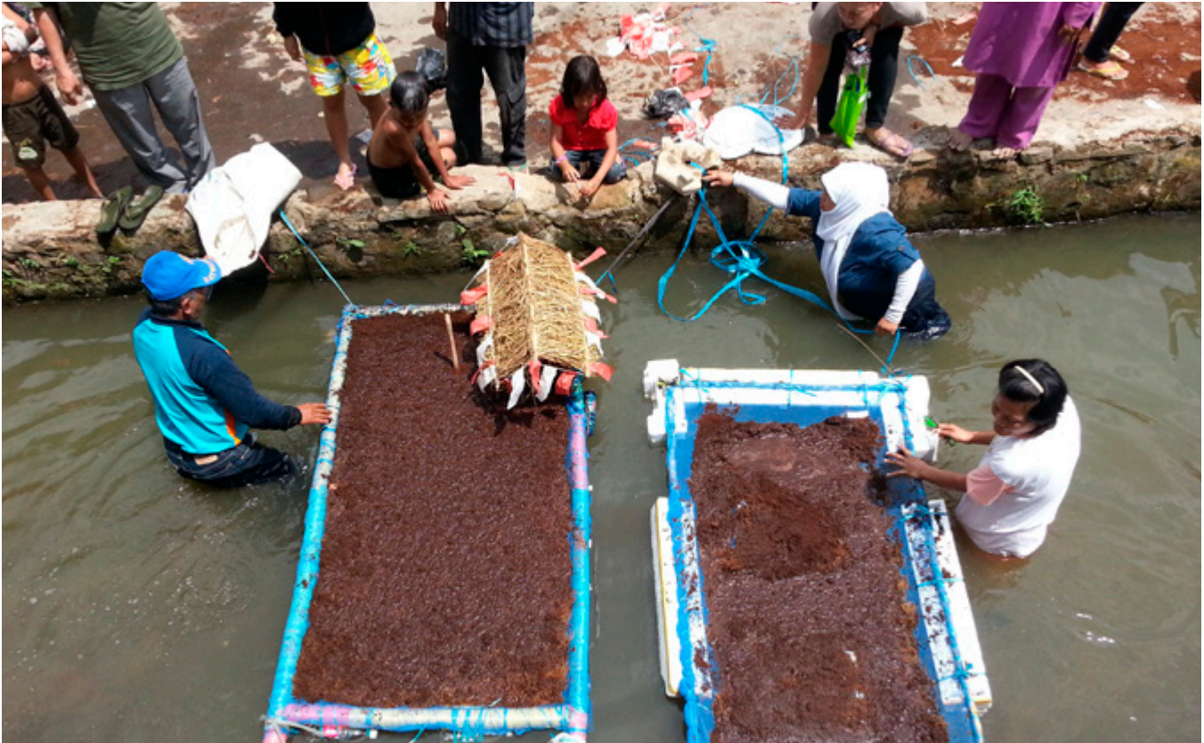
Construction of Floating Treatment Wetlands by the local community
