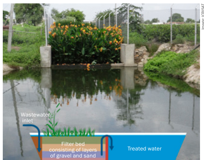
Constructed wetlands are one of the most cost-effective solutions for treating wastewater at community level
