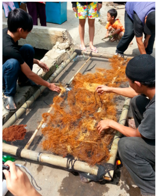
Construction of Floating Treatment Wetlands by the local community
