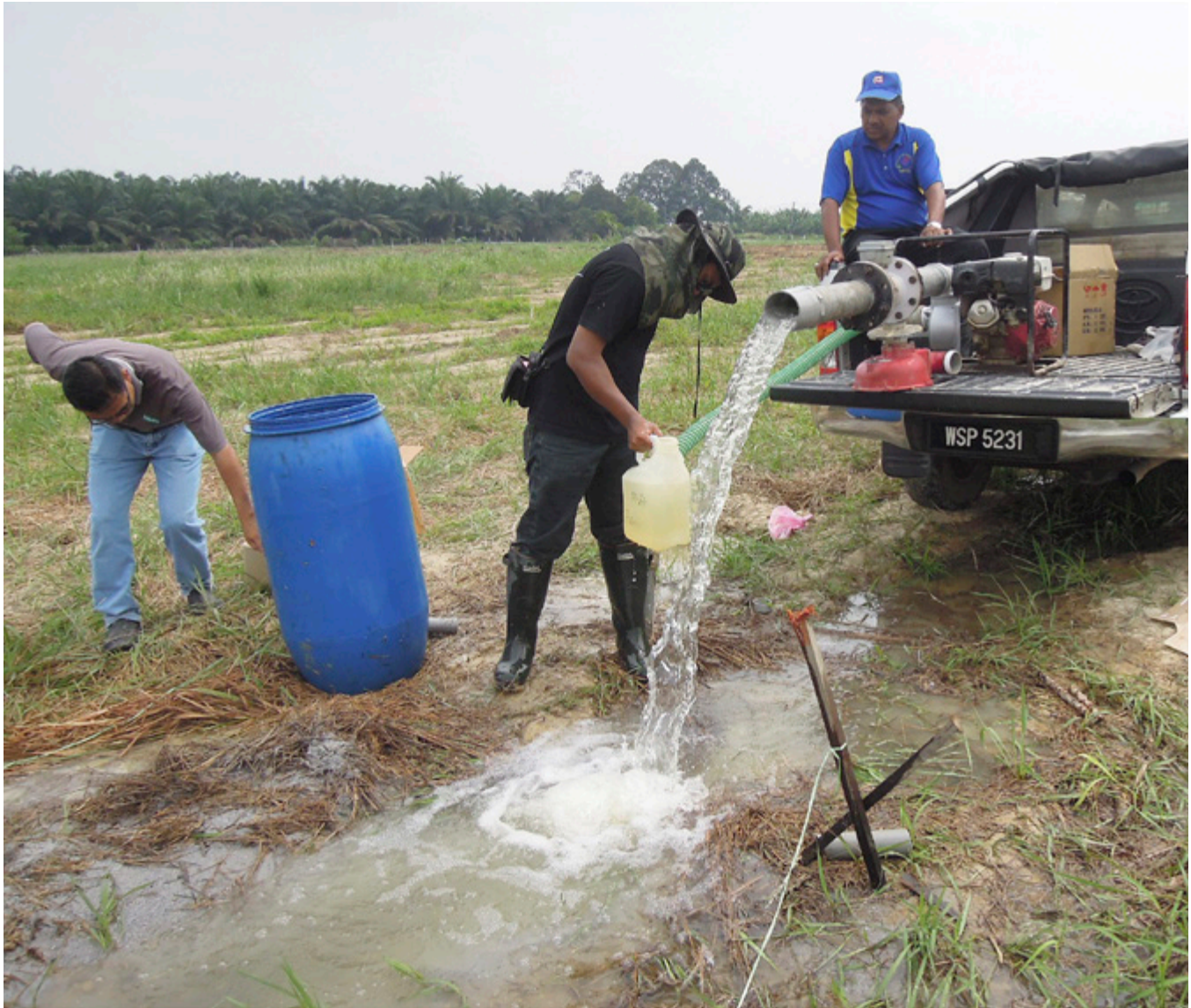
Fig. 4: Construction and testing of a shallow tube well for a small scale irrigation project
