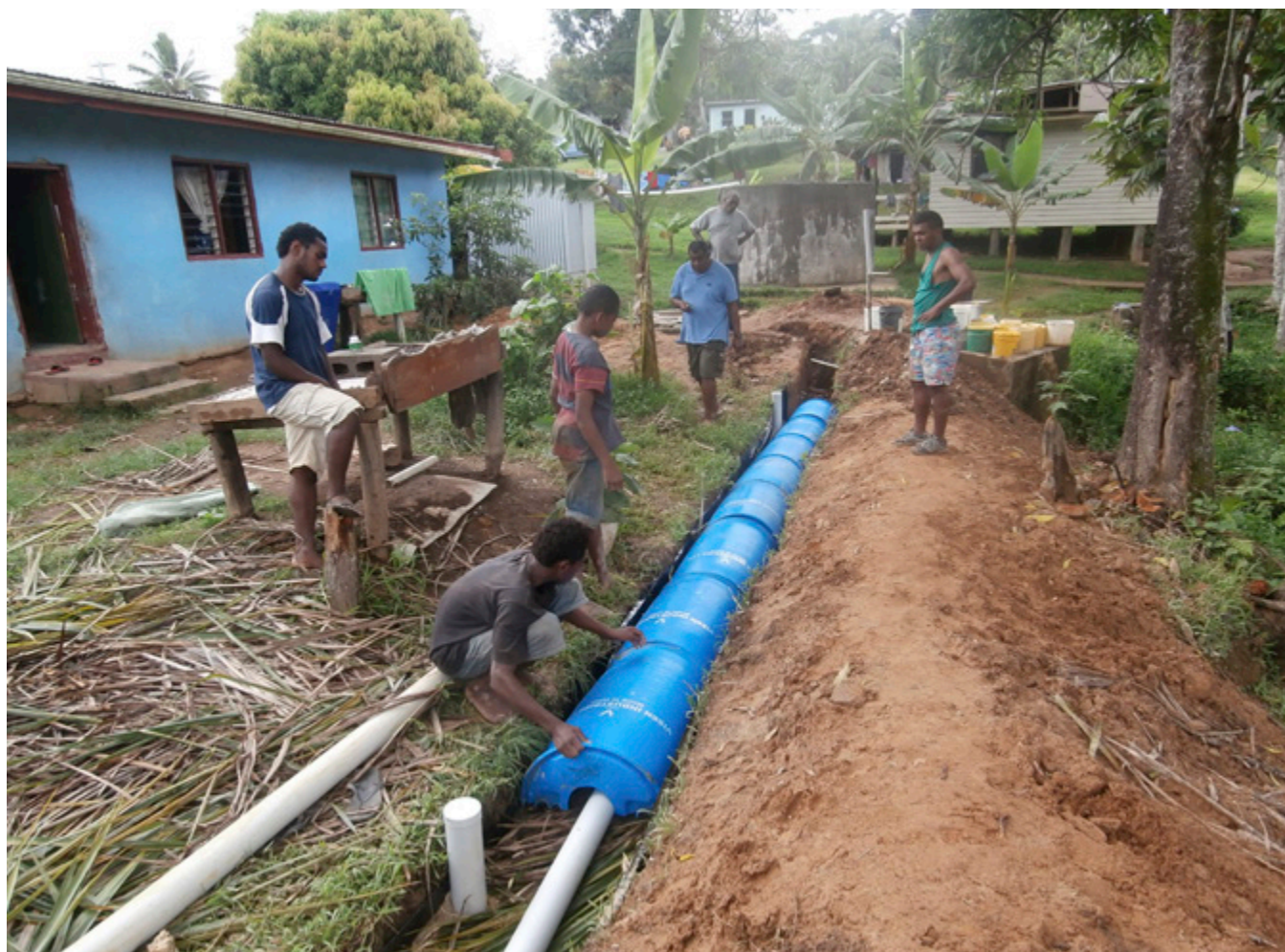
Constructing a sand filtration trench for land application of septic tank effluent in Bavu village, Fiji
