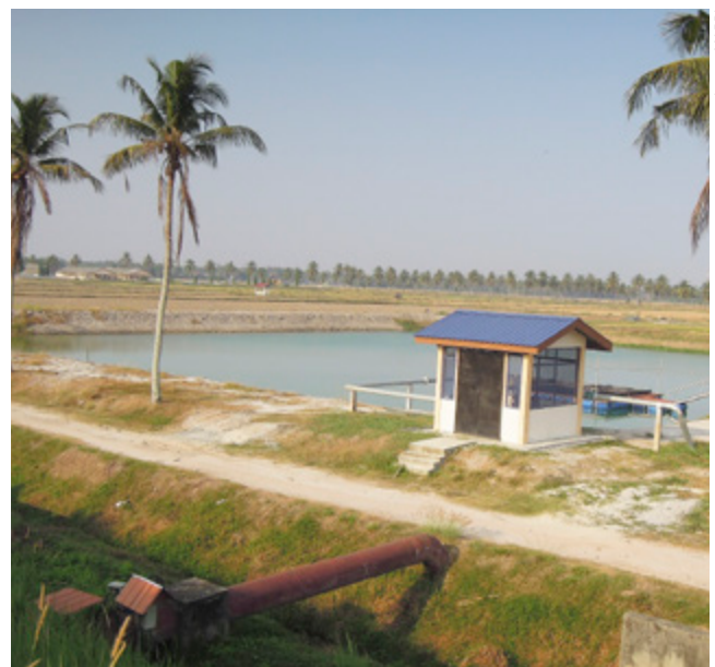
Fig. 2: Storage pond and pump house used in a tail water recovery project
