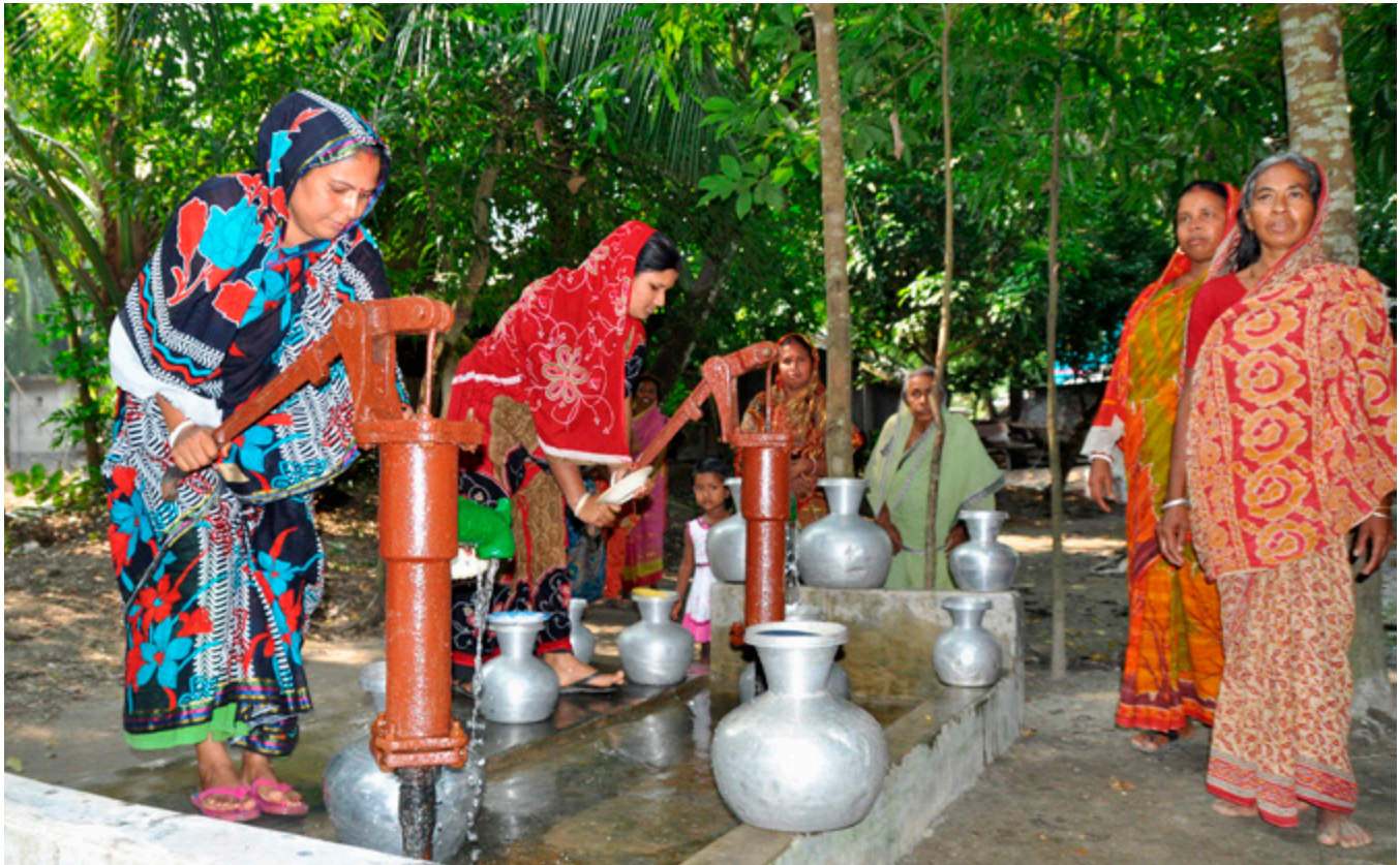
Double headed tubewell, an innovative transformation of a traditional deep tubewell by BRAC WASH in water-scarce areas of Bangladesh
