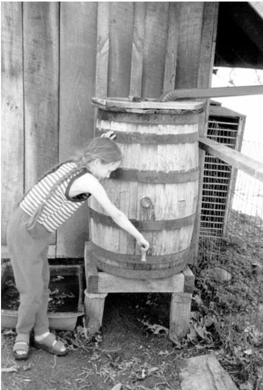
Phoebe demonstrating a simple rain water collection system used for watering chickens.
