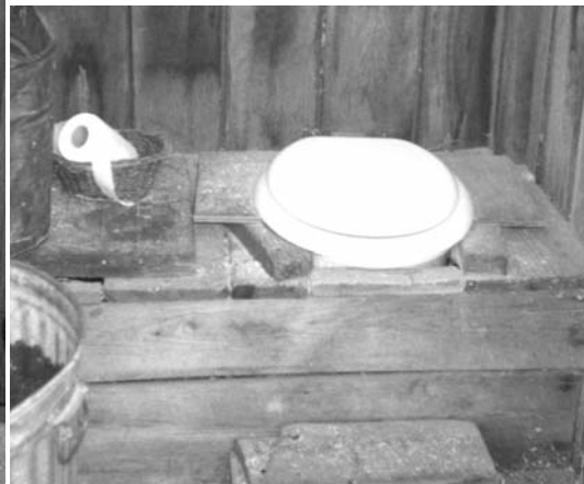
SAWDUST TOILET IN "OUTHOUSE" ▲
