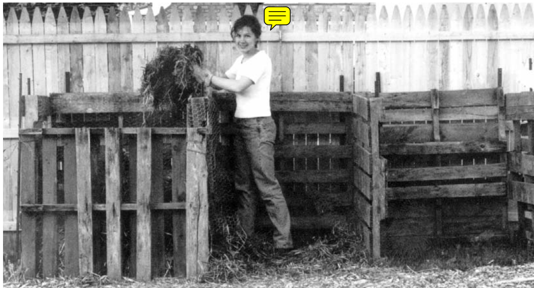
Newly constructed three-chambered compost bins made from pallets. The center chamber stores cover materials. This style compost bin costs practically nothing and can be erected in a short period of time. Photo by David Lott
