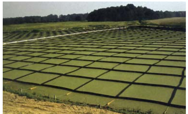
Photograph 5: A high density polyethylene grid system is used for duckweed stabilisation on the water surface in the shown duckweed-based polishing lagoon in the USA. It receives 500 m 3 /d of combined municipal, septic and industrial wastes after pretreatment in an aerated lagoon. (Photograph: Lemna Corp. 1994).
