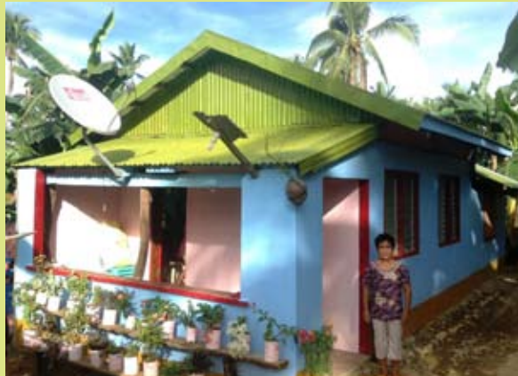
Households with “minor damage” received $423 to rebuild their homes.
