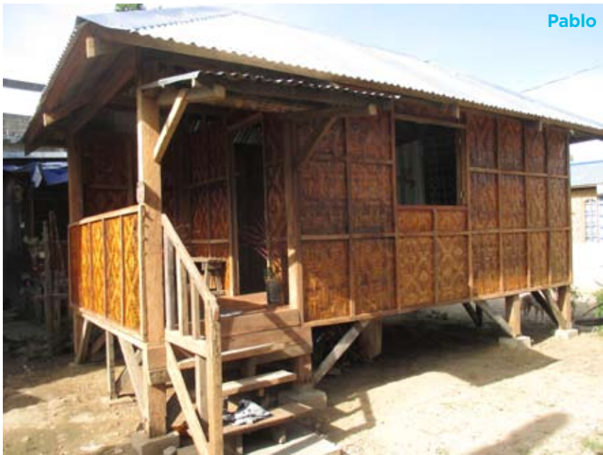
Left: The Pablo style (named after Typhoon Pablo which hit the island of Mindanao in 2012) is elevated 0.6 meters above the ground with a concrete footing and uses woven bamboo mats (known locally as amakan ) for walling.
