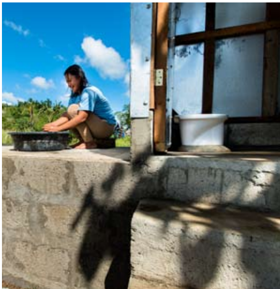
Left: The Type 6 toilet and septic tank is for households whose groundwater level is higher than 0.65 meters from the natural ground.
