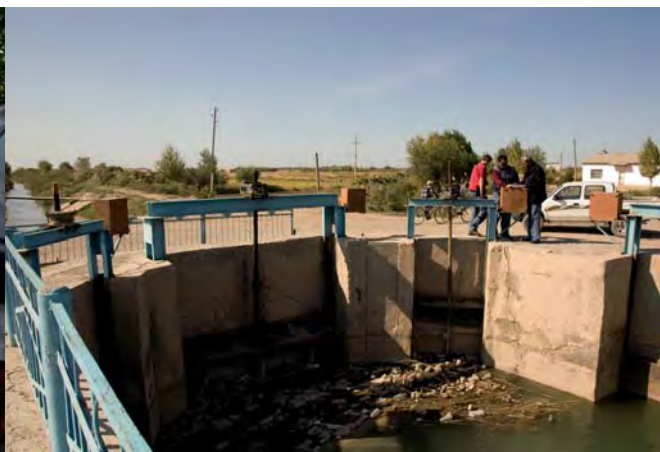
An irrigation channel with distribution structure
