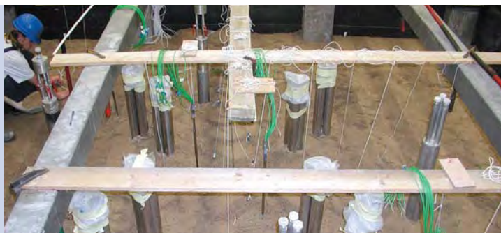
Heat lances and soil gas suction level being installed in the large tank
