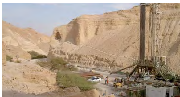
Test drilling for a well in the Judean desert near the Dead Sea as part of a research project
