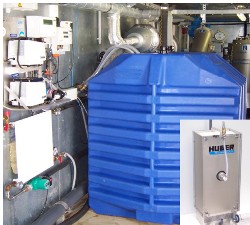
Figure 8: Photo and technical data of the HUBER GreyUse® unit
