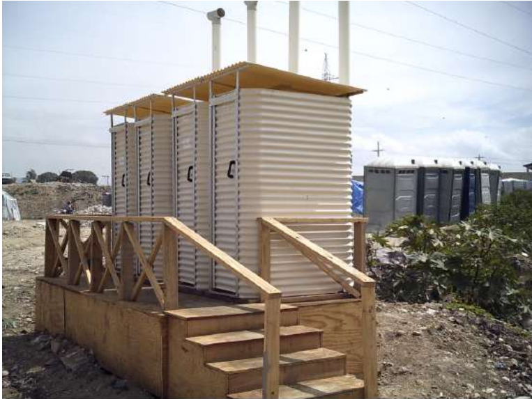
Haiti – raised latrines using plastic tank for containment of excreta
