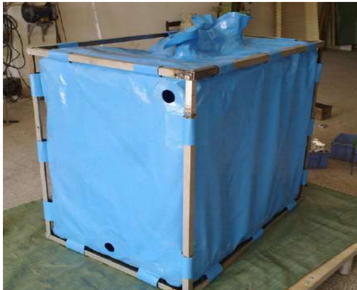
Haiti – raised latrines using plastic tank for containment of excreta
