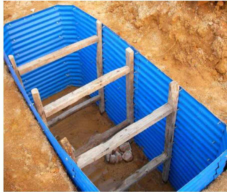
Trench pit liner - propped
