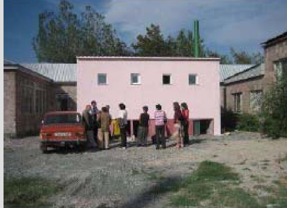
Figure 3: the new ecosan toilet facility for 350 pupils (source AWHHE)
