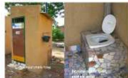
Fig. 3: Outside and inside views of a single vault UDDT in Ouagadougou (with urine diversion seat).
