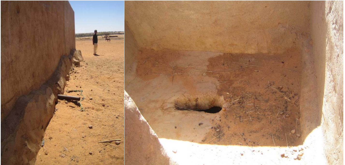
Touloum refugee camp: collective latrines with liquid diversion; exterior and interior
