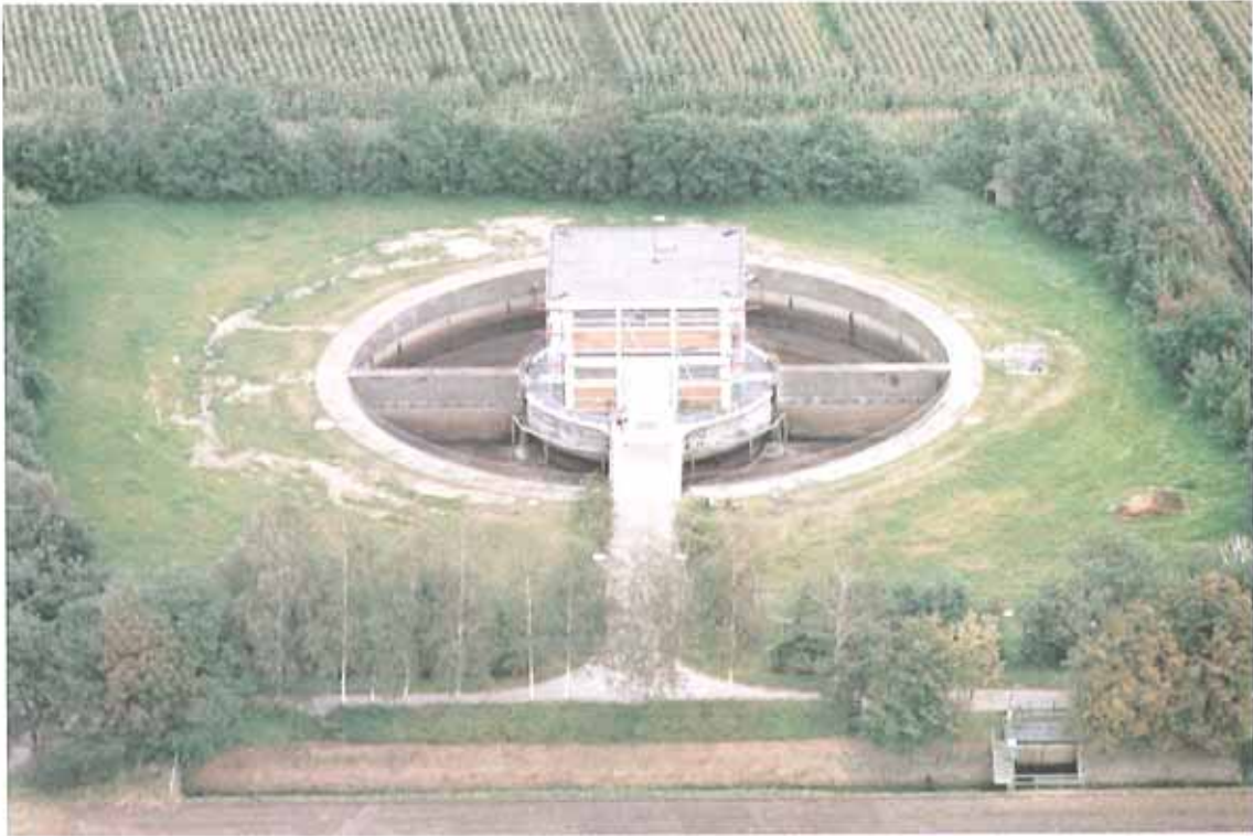
Main pumping station IV
