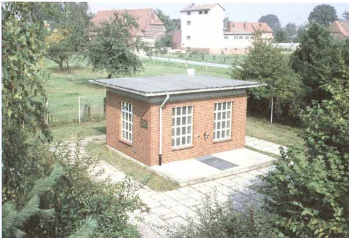
Local pumping station
