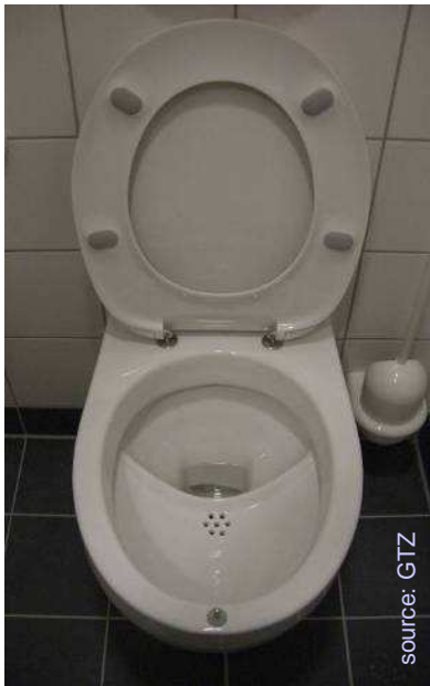
42 low flush urine separation toilets (1 L per urine flush, 6 L per faeces flush)
