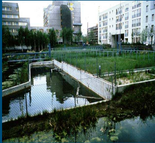
Local Water treatment in Berlin
