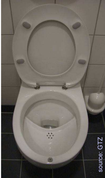
urine separation toilet
