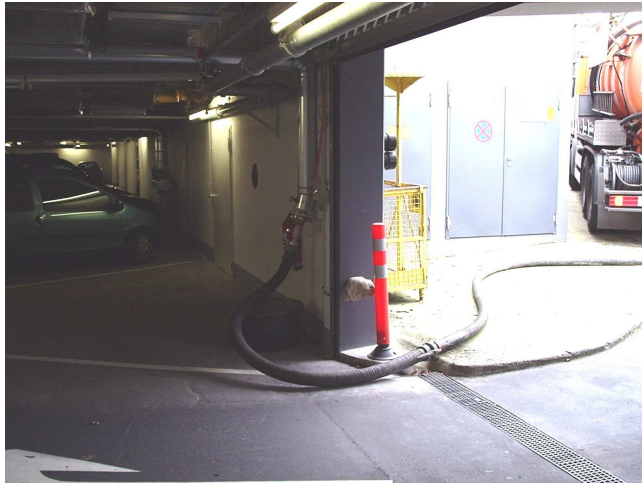
pump truck connection to docking station
