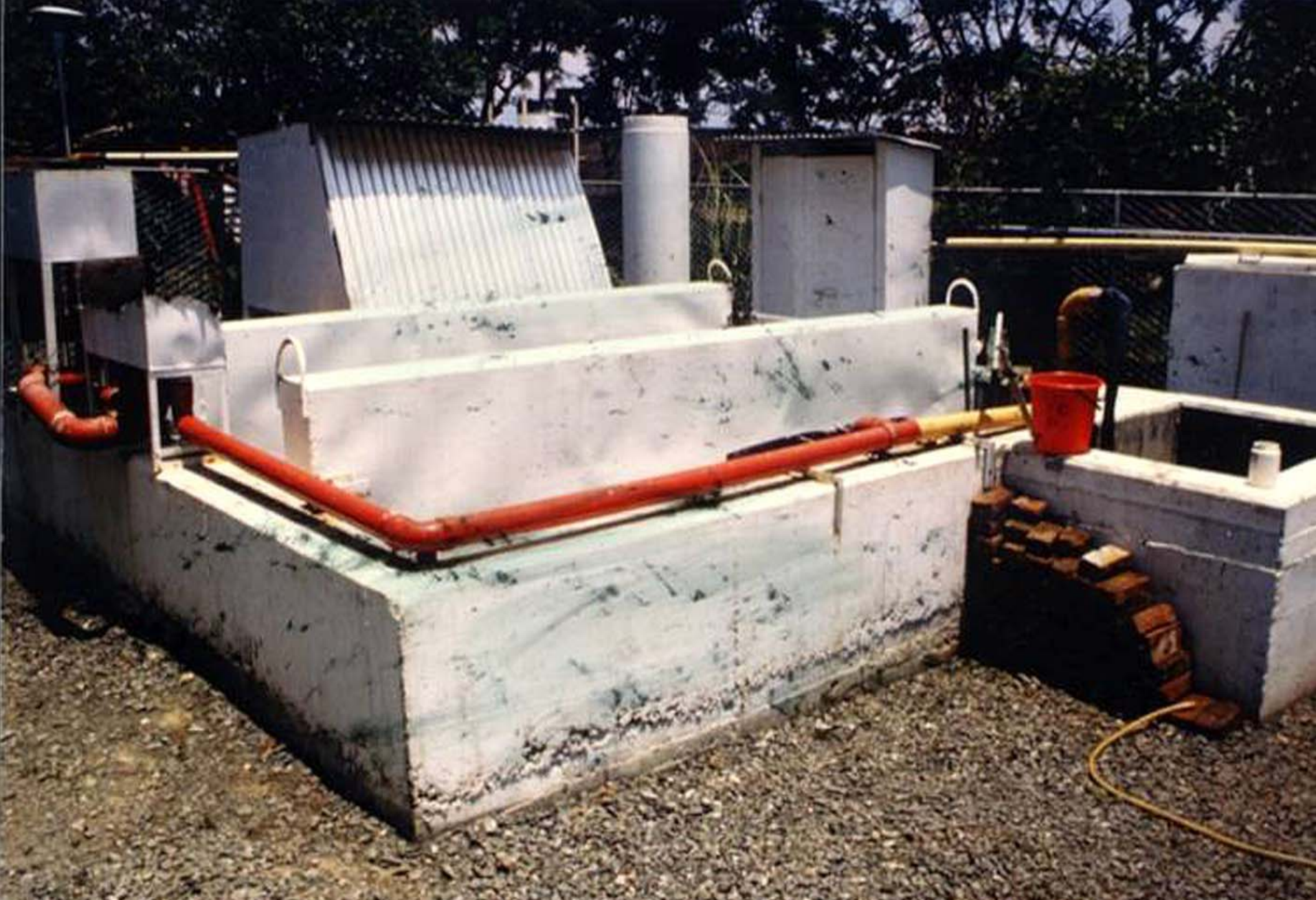
The 64 m 3 demonstration UASB-plant in Cali Colombia (1983-1989)
