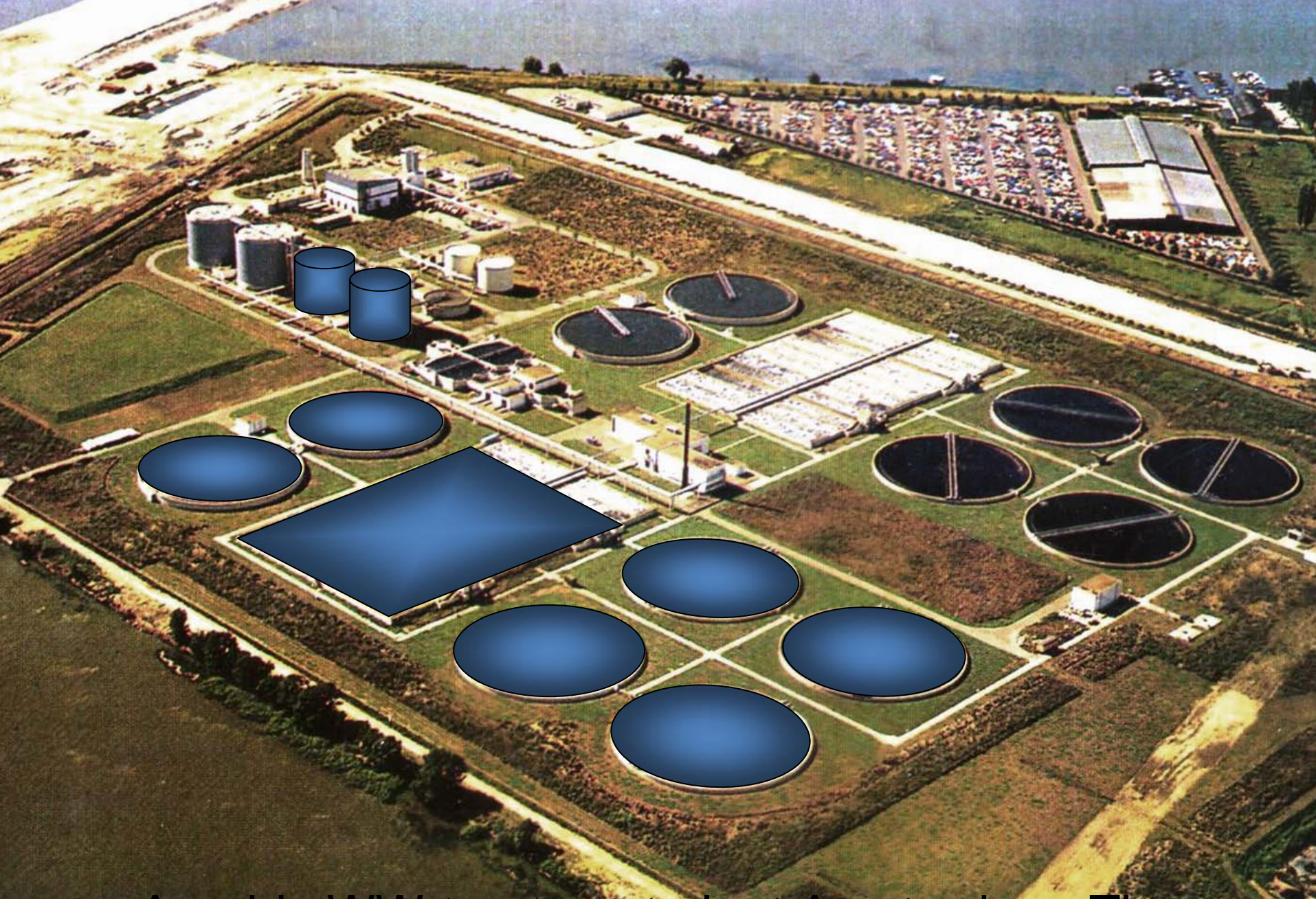
Aerobic WW-treatment plant Amsterdam, The Netherlands
