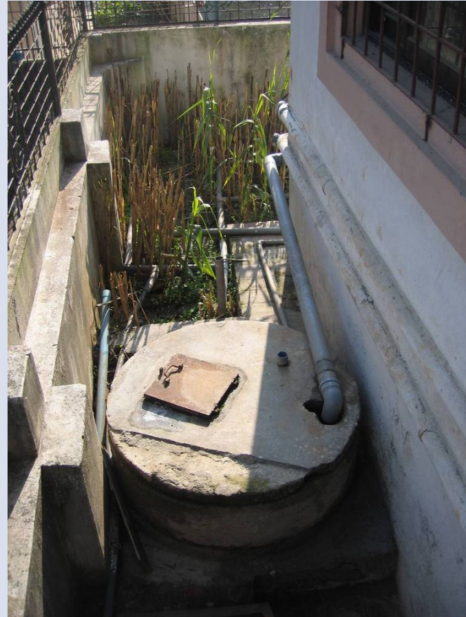
Dug well for groundwater collection and recharge
