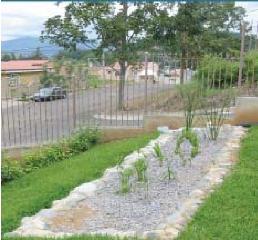
Grey water treatment
