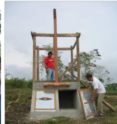
City provides for the sub-structure as key strategy
