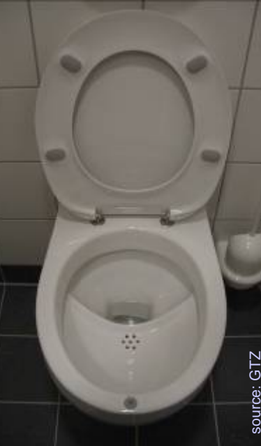
urine separation toilet
