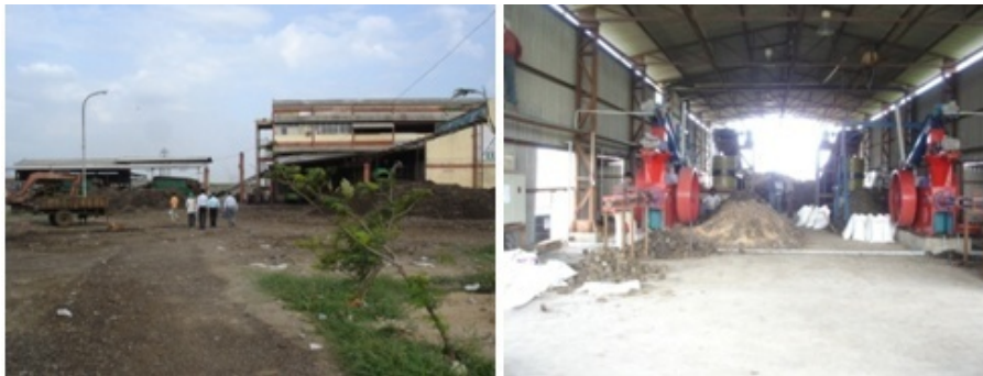
Figure 41 MSW Processing Facilities at Excel Industries (left) and UPL Djai Power Ltd. (right)
