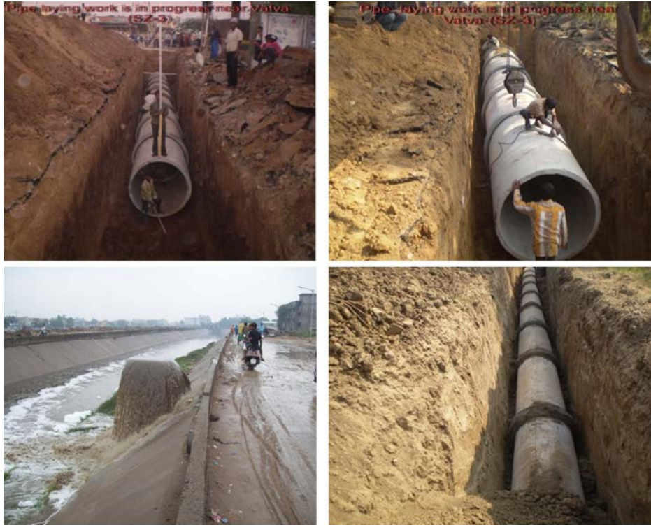
Figure 15 New Pipelines Laying
