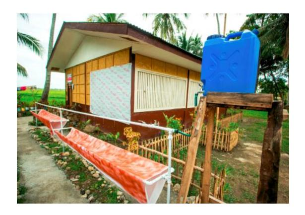
2013 Modular punched GI pipe with flexible external tank
