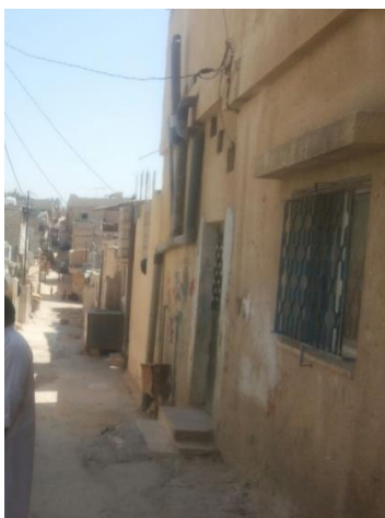
Ground water tank in Jarash camp
