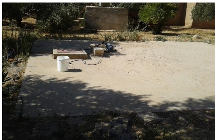
Ground water tank in Kharja
