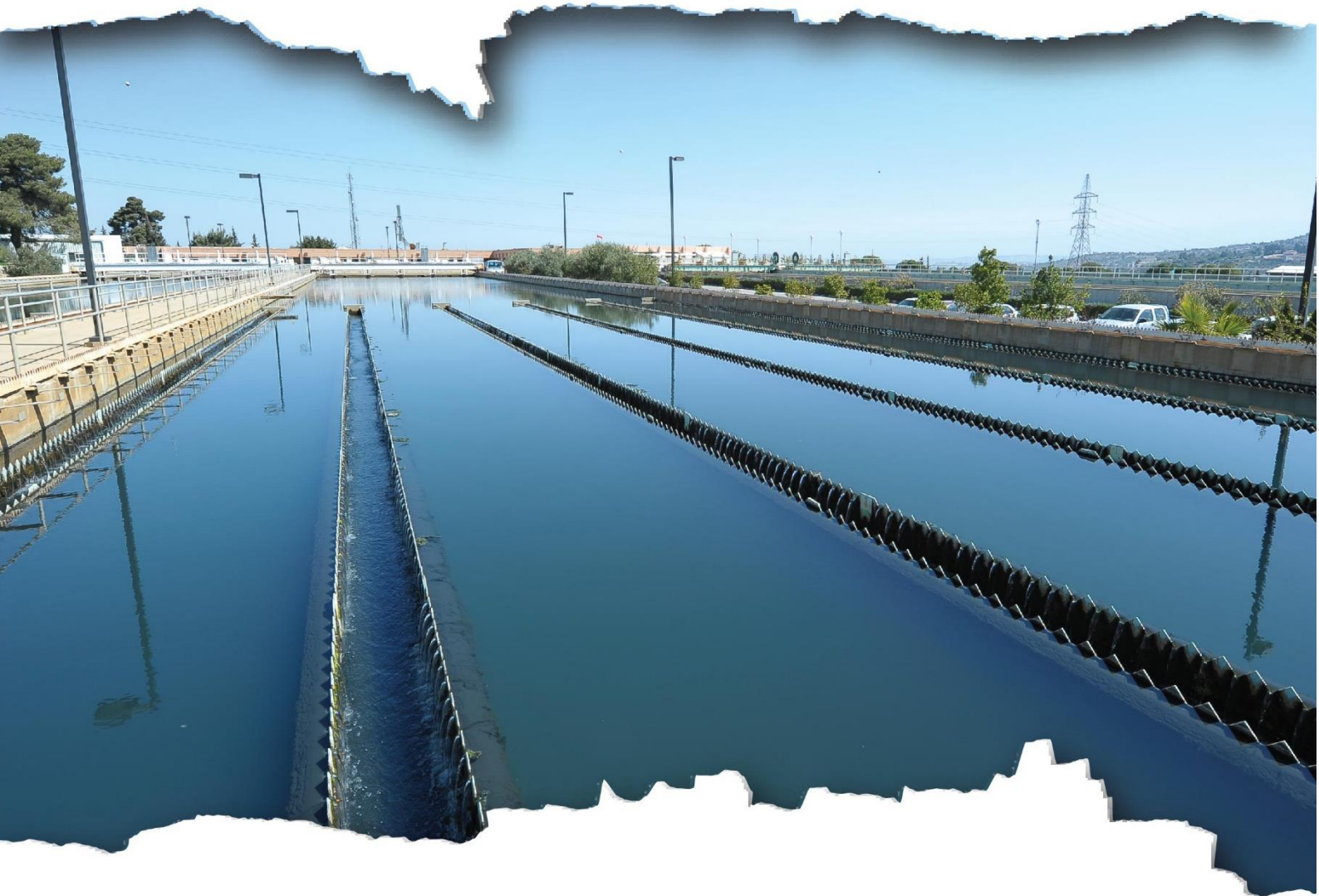
ZAI WTP - Jordan
