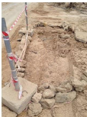
Network pipe laying in Al Hosson village
