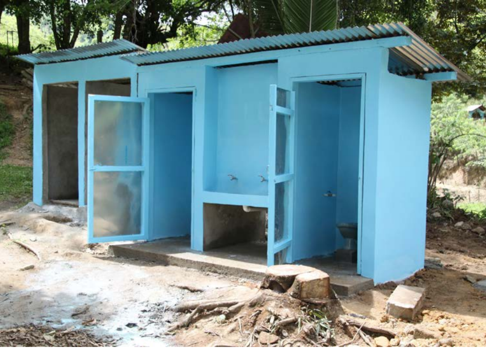
School toilets with a handwashing station.
