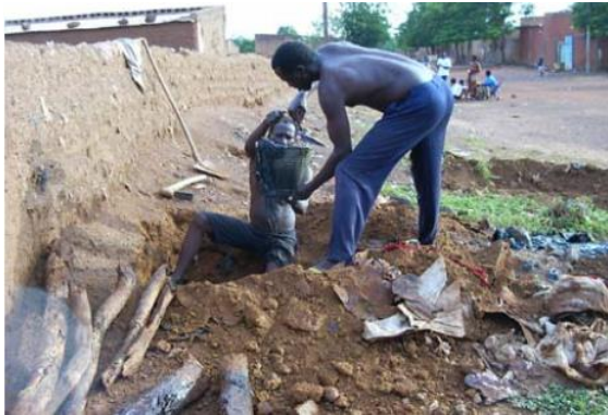
Figure 8: Manual operators emptying a pit in Ouahigouya (credit: Koanda Halidou, 2006)
