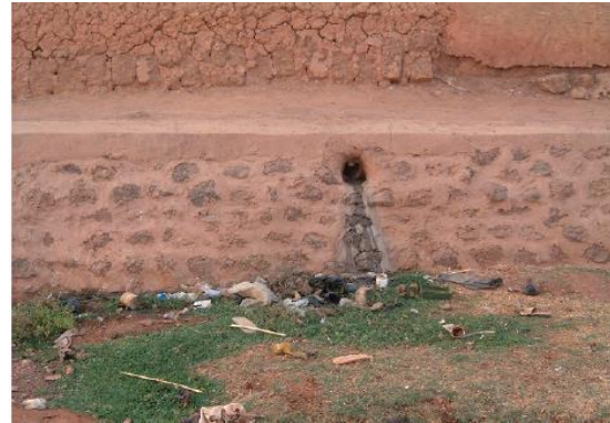
Figure 9: Shower connected to an open channel in the street (credit: Koanda Halidou, 2006)
