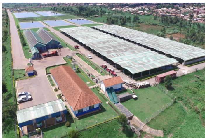
Aerial view of Lubigi Waste Water and Faecal Sludge Treatment Plant (WW&FSTP) producing 300 tonnes per month of soil amendment, a marketable product sold to farmers (source: presentation by Eng. Oyuru)
