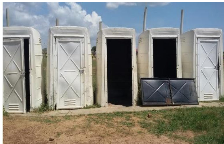
Figure 10: Latrines in Gulu and Katakwi
