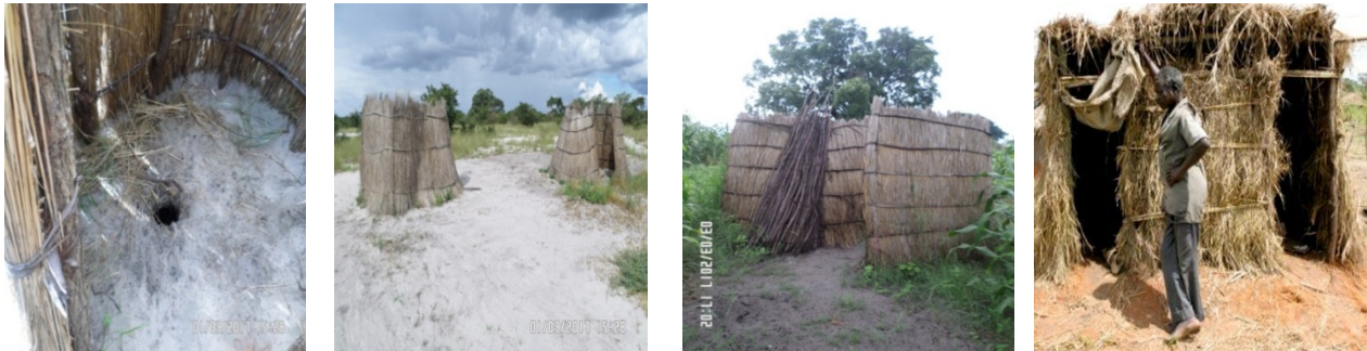
The type toilets used by school pupils and teachers at both primary schools, pictured by Patrick Maboshe.
